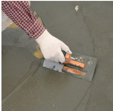
Resurfaces Spalled & Pitted Concrete
