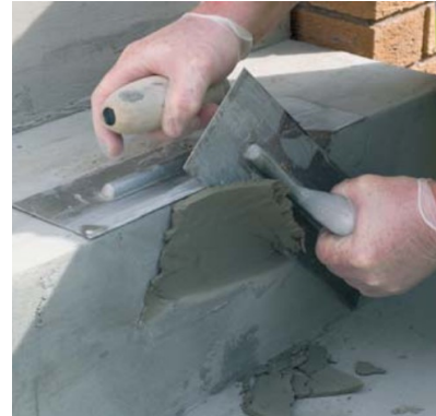
Vertical and Overhead Patching & Repairs up to 2"
