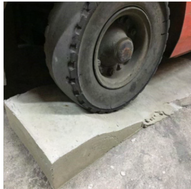
Horizontal Patching & Repairs up to 6"
